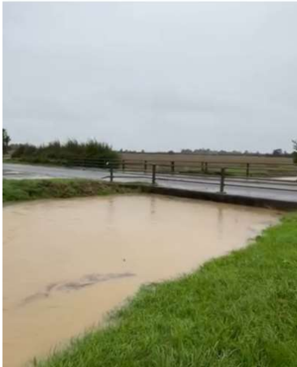
The bridge at the turn to Broxholme from the A1500
